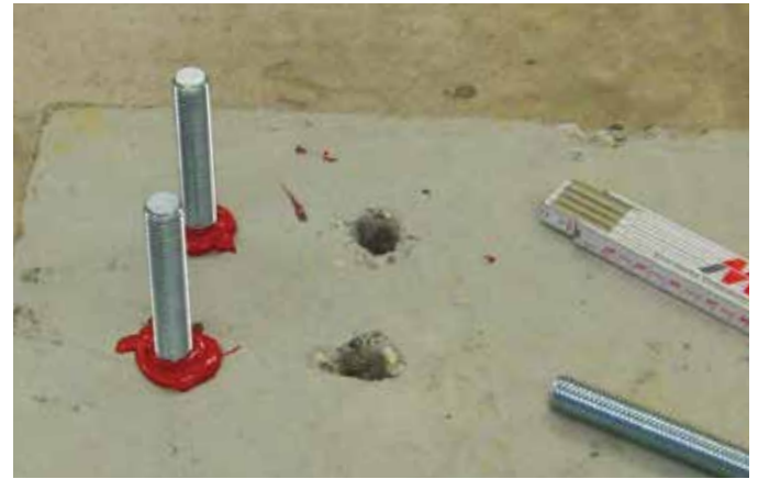
Threaded Stud VM-A 1 meter length, to be cut to the required length
